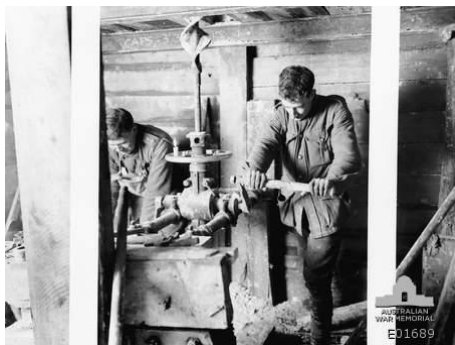
Men of 3ATC utilising a vertical wombat borer to provide ventilation at Cite St Pierre, Lens
