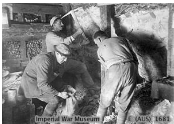
Men of 3rd Australian Tunnelling Company excavating a chamber in the chalk in the Hulluch subway
